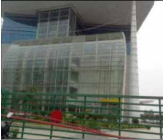
Front view of Building
