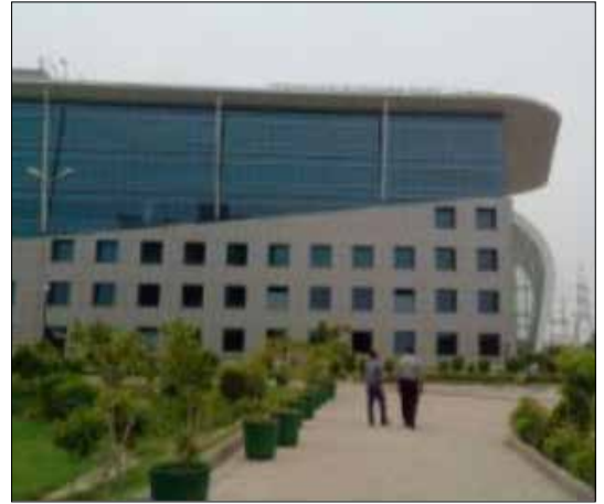
Side view of Building
